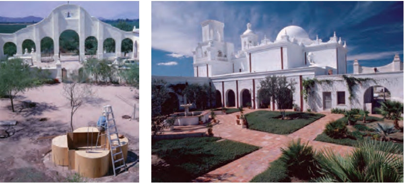
[Image 41] (lower left) A circa 1968 photo shows a mold being prepared in the Patio to pour concrete for the new fountain. Previously, the Patio, or courtyard, had served more utilitarian functions. (University of Arizona Special Collections Library)
