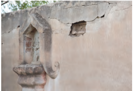
[Image 81] Some lower priority areas and features, such as the atrium and cemetery walls, show signs of deferred maintenance, such as cracking and delamination.
