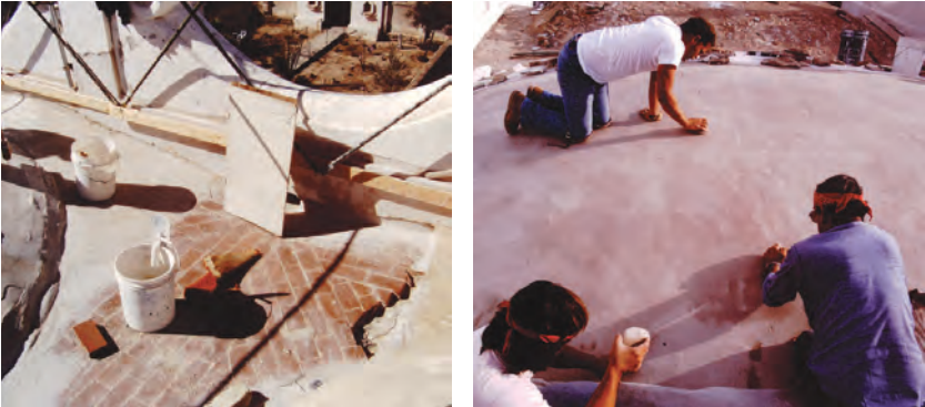
[Image 44] (left) Lower-lying areas of the roof were repaired with harder, higher-fired modern brick, to encourage water runoff and drainage. (Robert Vint)
