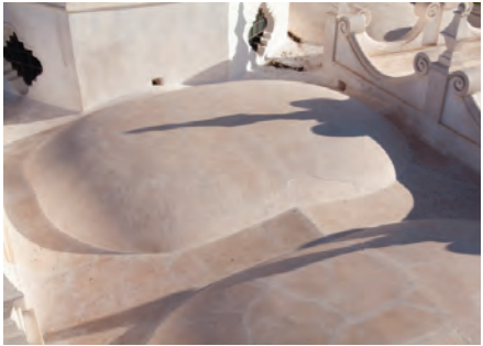
[Image 80] Webbed cracking in the render of the roof vaults is caused by natural cycles of expansion and contraction. Despite the inclusion of expansion joints in the surface render, cracking has persisted and some delamination has occurred.
