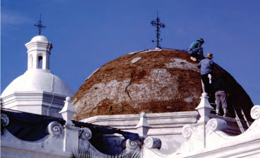
[Image 43] After a large piece of plaster fell from the ceiling in 1989, it was determined that impermeable cement-based and synthetic coatings were accelerating the deterioration of the underlying brick and creating dangerous conditions inside the Mission. Beginning with the roof's dome and vaults, impermeable cement-based coatings were systematically removed, the substrate repaired, and the whole re-coated with a more compatible lime-based mixture. Removal of the existing coatings revealed large, deep cracks in the central dome. Work was supported by numerous grants and has been ongoing for more than 30 years. All images on this page were taken circa 1993 by architect Robert Vint, who oversaw this work.
