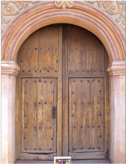
[Image 82] The original yellow pine doors are still in place, though they have deteriorated from exposure to the elements. They have never undergone conservation treatment.
