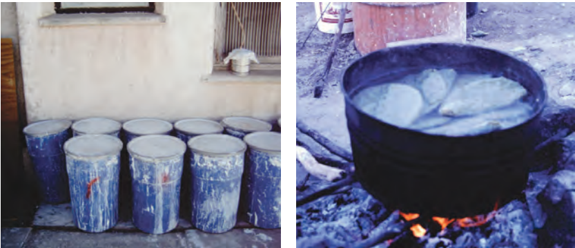
[Image 46] (left) Lime putty slaking in plastic barrels on site. Slaking the lime for weeks or even months in advance improves its workability. (Robert Vint)
