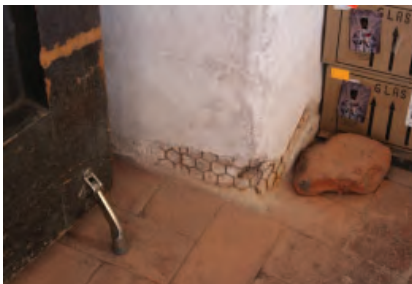
[Image 75] Exposed reinforcement wire beneath cement-based render in the South Convento Wing.
