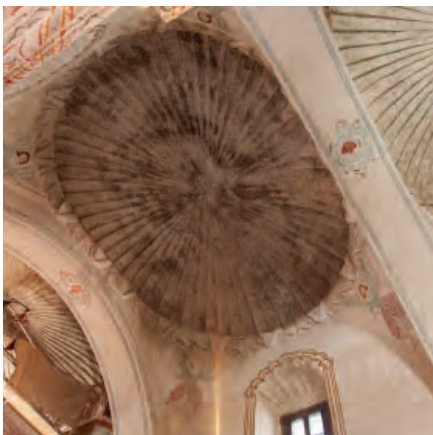
[Image 78] Evidence of prior water damage is present on some of the vaults, but the current extent and patterns of infiltration and moisture movement are not well understood.
