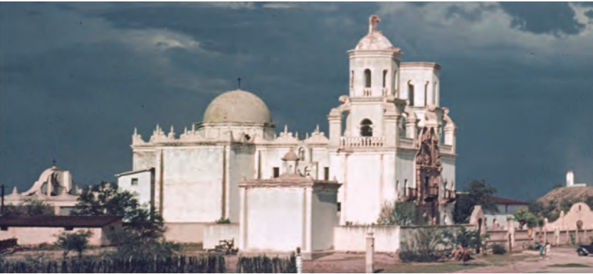
[Image 38] View of the Mission circa 1939 showing lightning damage to the West Tower lantern. The central dome also appears darker than other parts of the building, suggesting that a different coating may have been applied to it, perhaps in an attempt to limit water infiltration. (University of Arizona Special Collections Library)
