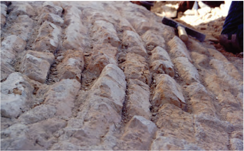
[Image 48] Due to decades of deterioration from water infiltration, some portions of the low-fired brick comprising the vaults, dome, and walls have substantially eroded, as seen in this photograph. In other areas the substrate was very much intact and traces of well-adhered original plaster still remained and were left in place. (Robert Vint)
