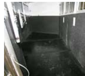
New composite rubber wall lining in horse area
