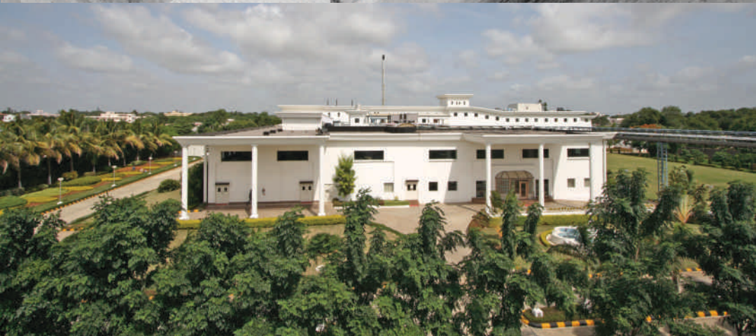
The blueprint (Top) of the factory of Shantha Biotechnics and the factory building (Bottom) (Photo Courtesy: K. Varapasad Reddy)
