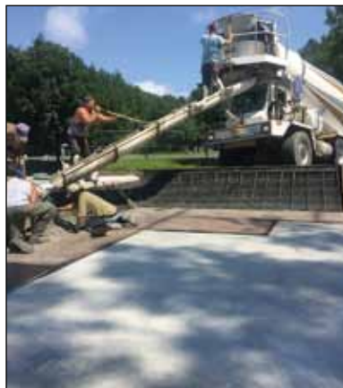
Pouring cement for the updated park
