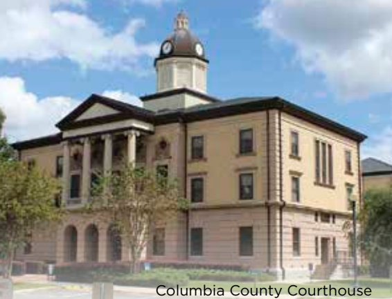
Columbia County Courthouse
