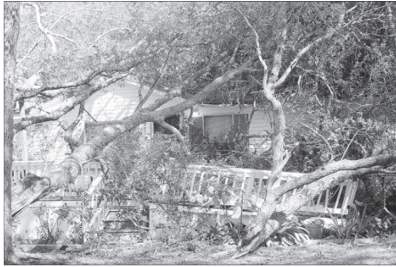
A large tree collapsed the front deck of Ava Casto's home on Tuesday night. "I was shocked," Casto said.
