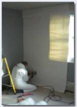
Spaceloft's thin profile offers the same R-value as traditional thick insulation with minimum interior space lost – especially beneficial to solid masonry building retrofits.
