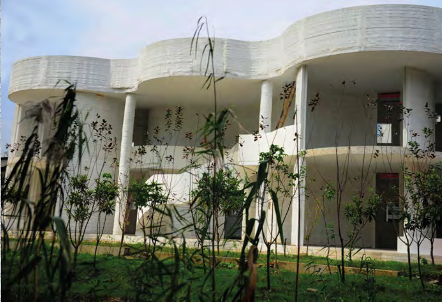
A 3D-printed house at Suzhou Industrial Park in Jiangsu Province, China
