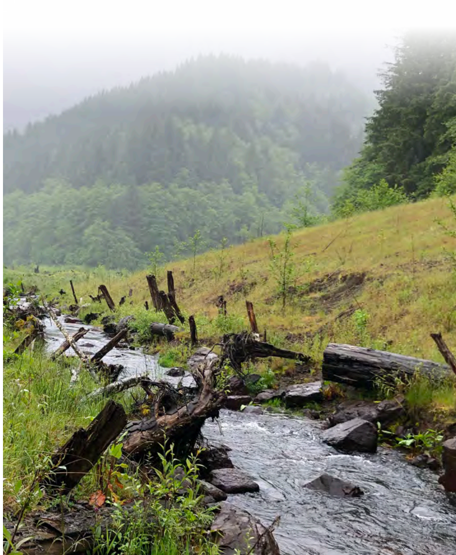
Fawcett Creek channel through breached dam site.
