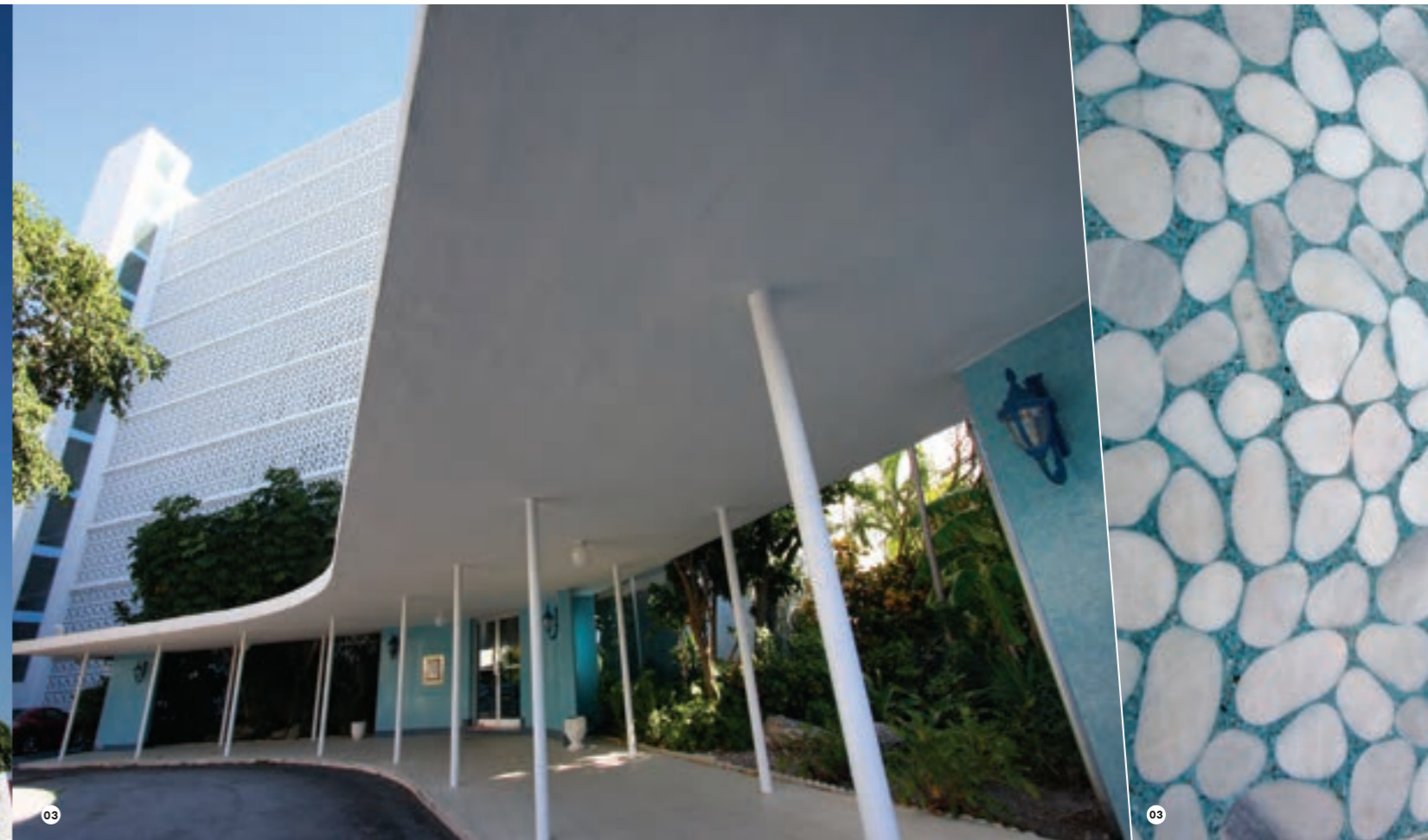
A sweeping boomerang-shaped porte cochere balanced on beanpoles, turquoise and white mosaic tile, and breezeways inventively masked with miles of screen block are a breathtaking combination at the Mediterranean, designed in 1957 by A. Herbert Mathes.
