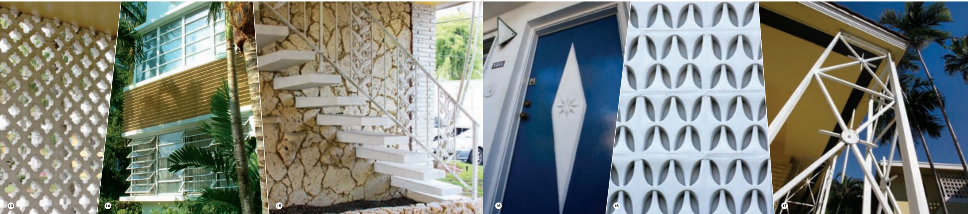
FROM LEFT Decorative screen block, bands of awning windows, a floating staircase and rustic stone-clad wall are common elements found in BHI's MiMo buildings.
