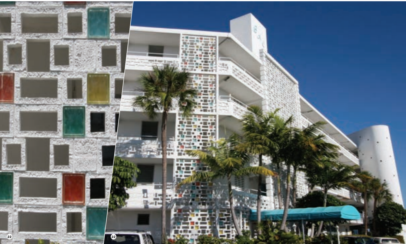
By inserting colored glass rectangles into white cast-concrete screen block, Charles McKirahan gave his Bay Harbor Continental (1958) a playful appearance and a stylish shield from the sun. Stairwells and elevator shafts are artfully hidden too.
