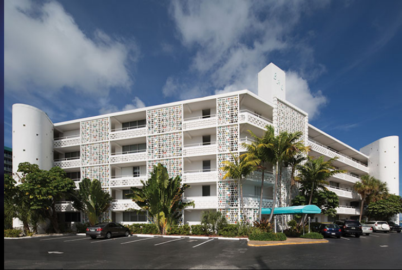
Tray balconies and breezblock walls studded with multi-colored glass block are just two of McKirahan's signature treatments at the Bay Harbor Continental, built in 1958.
