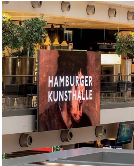
Digital signage installed at Hamburg Airport incorporates self-activating fire extinguishers.
