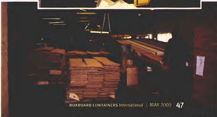
West Indies Paper Products installed a used, two-color, 60-in.-x-80-in. Ward rotary diecutter (top) to produce more sophisticated boxes. Its 85-in. Langston corrugator produces B- and C-flute corrugated.
