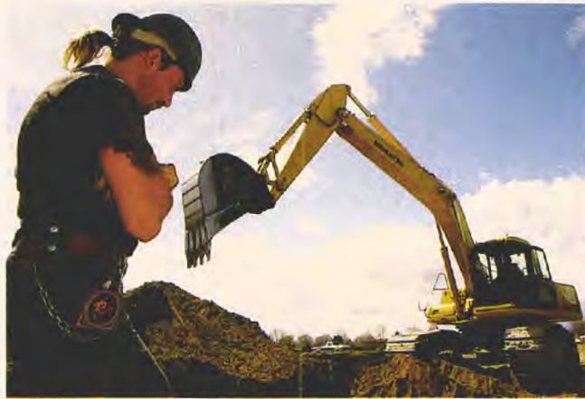
Building the Forest Park subdivision in Billings
