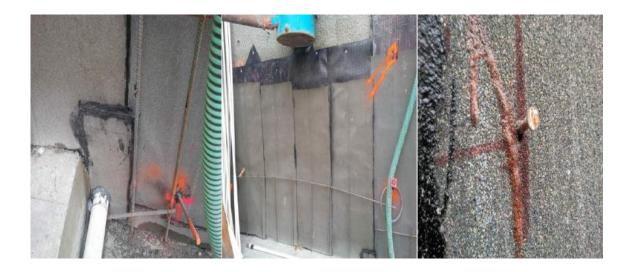
The number of seams in this membrane are even more numerous. That in turn increases the risk for waterproofing failure.
