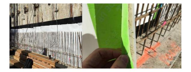
What we're looking at is a pre-applied composite membrane that's been installed in preparation for blindside shotcrete foundation walls.
