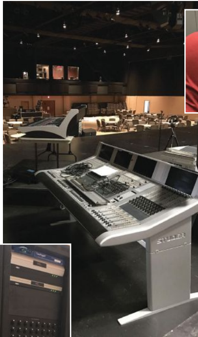
Among the items that were installed at Granger included a LAWO digital 8 analog-to-IP interface race unit (left). A volunteer (top) helped to install the equipment in December 2016. The Lawo mc 2 56 console is shown (center) prior to the completion of the install.
