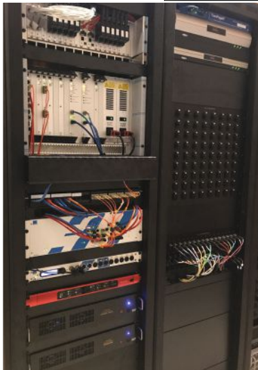
Among the items that were installed at Granger included a LAWO digital 8 analog-to-IP interface race unit (left). A volunteer (top) helped to install the equipment in December 2016. The Lawo mc 2 56 console is shown (center) prior to the completion of the install.
