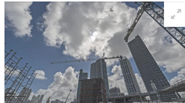
Construction in downtown Miami JOCK FISTICK
