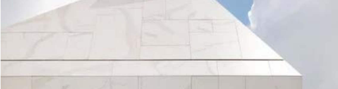
The porcelain tile cladding is a unique choice. "We thought we'd work with all the available off-the-shelf tile formats and mix them up in an interesting pattern. It really relied on having a little bit of adjustment in the installation."
