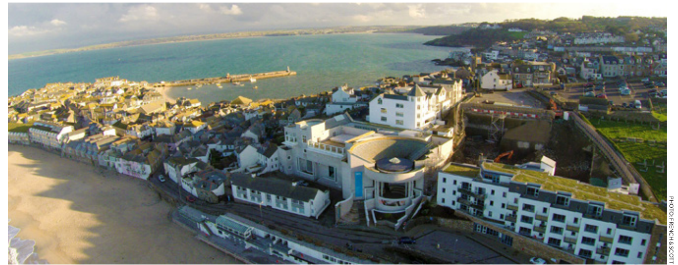
Aerial view of Tate St Ives from 2014 showing building work underway
