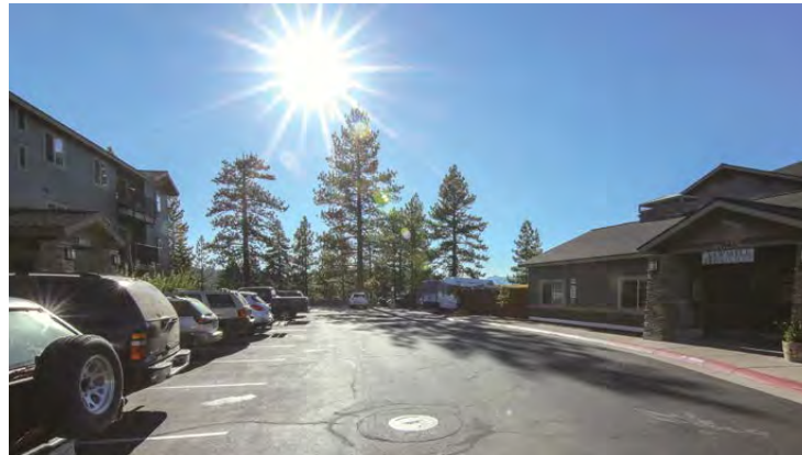
UP AND RUNNING AFFORDABLE RENTALS: Sawmill Heights is the only apartment complex located in Northstar and was built for employee housing. Photo by Jeremy Jensen/Moonshine Ink
