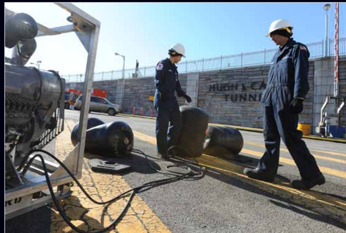
Petty Officer 2nd Class Sharina Lamonica and Petty Officer 3rd Class Brian Lamoria monitor a hydraulic prime mover and pumping equipment during dewatering operations at the tunnel in New York City, Nov. 9, 2012.
