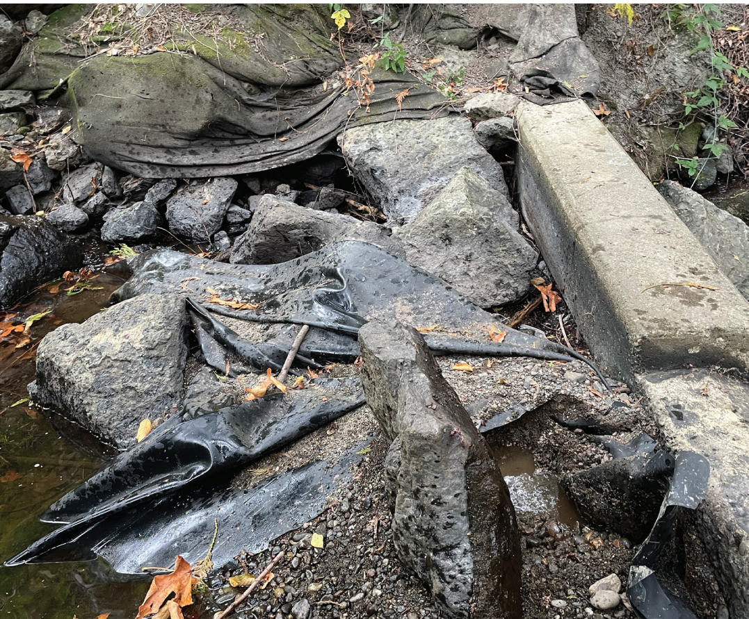
Springbrook Creek Weir during low flow conditions
