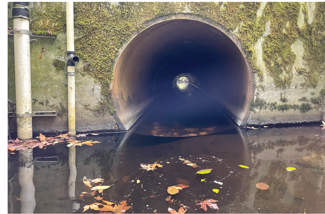
Culvert at Springbrook Creek
