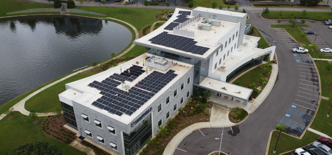
Sheffield Project Pictured Above
