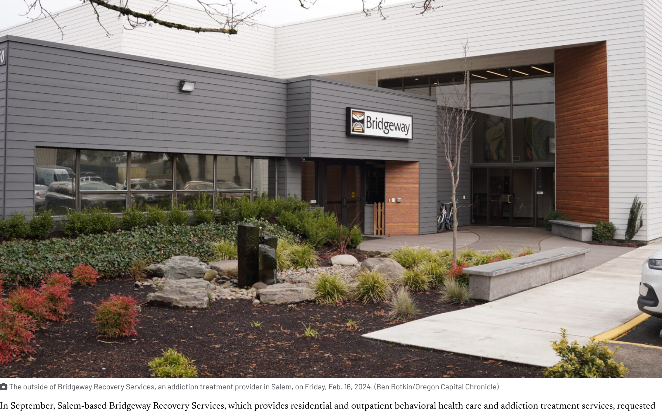
■ The outside of Bridgeway Recovery Services, an addiction treatment provider in Salem, on Friday, Feb. 16, 2024. (Ben Botkin/Oregon Capital Chronicle)
