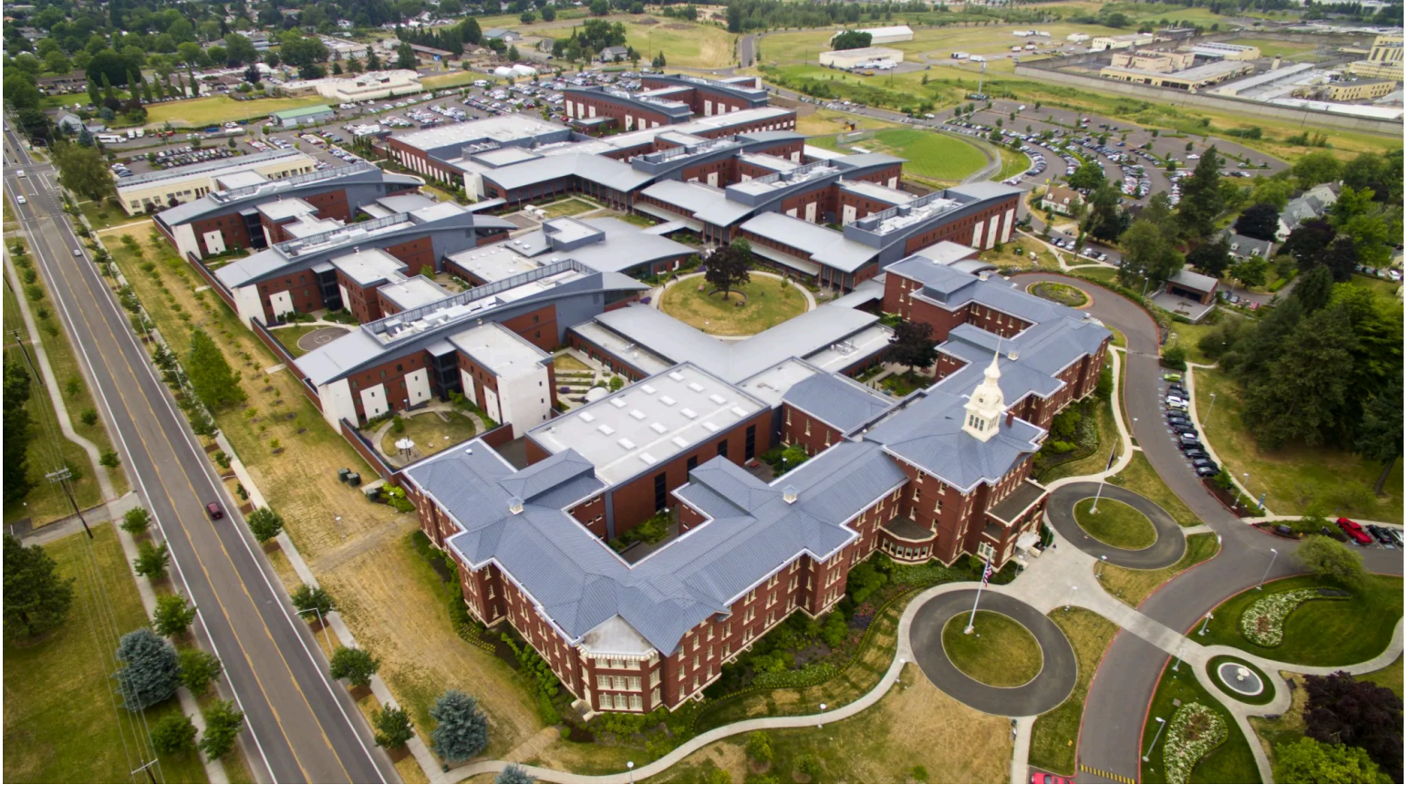
Oregon State Hospital, the state's psychiatric hospital, serves nearly 600 patients at its main Salem campus.
