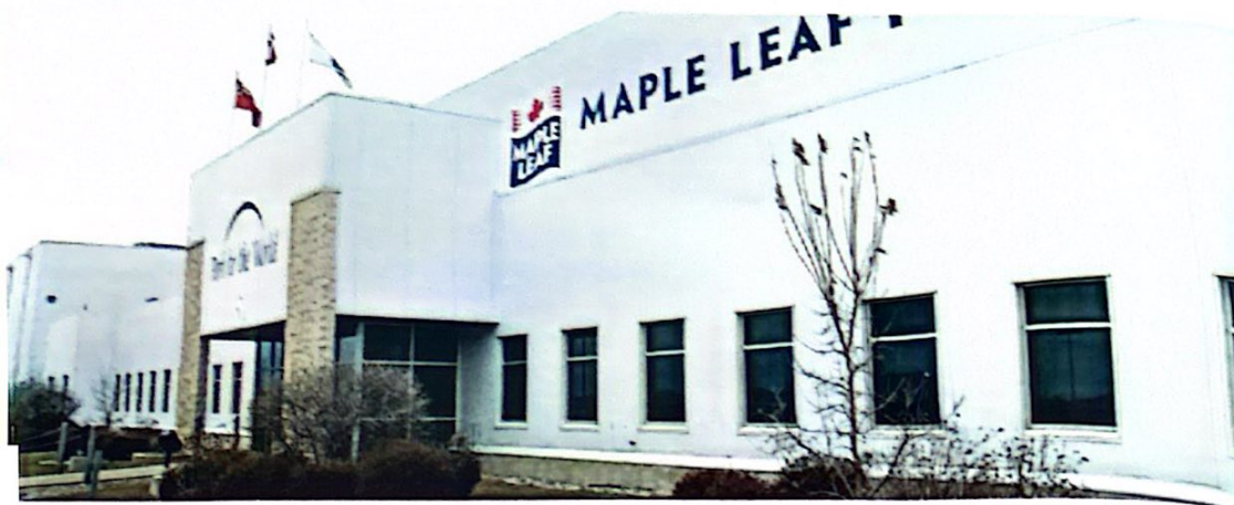
Maple Leaf's pork processing plant in Brandon, Manitoba is the largest facility of its kind in Canada.
