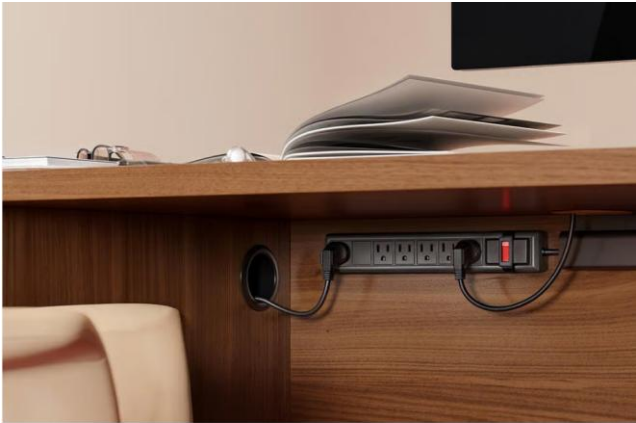
Power bars/strips and cable management
