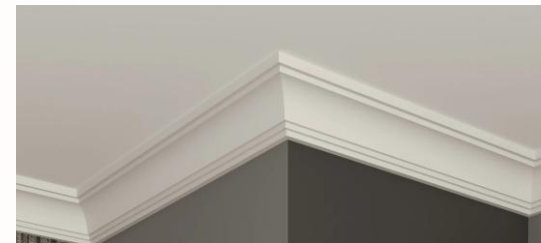
Ceiling Crown Molding
