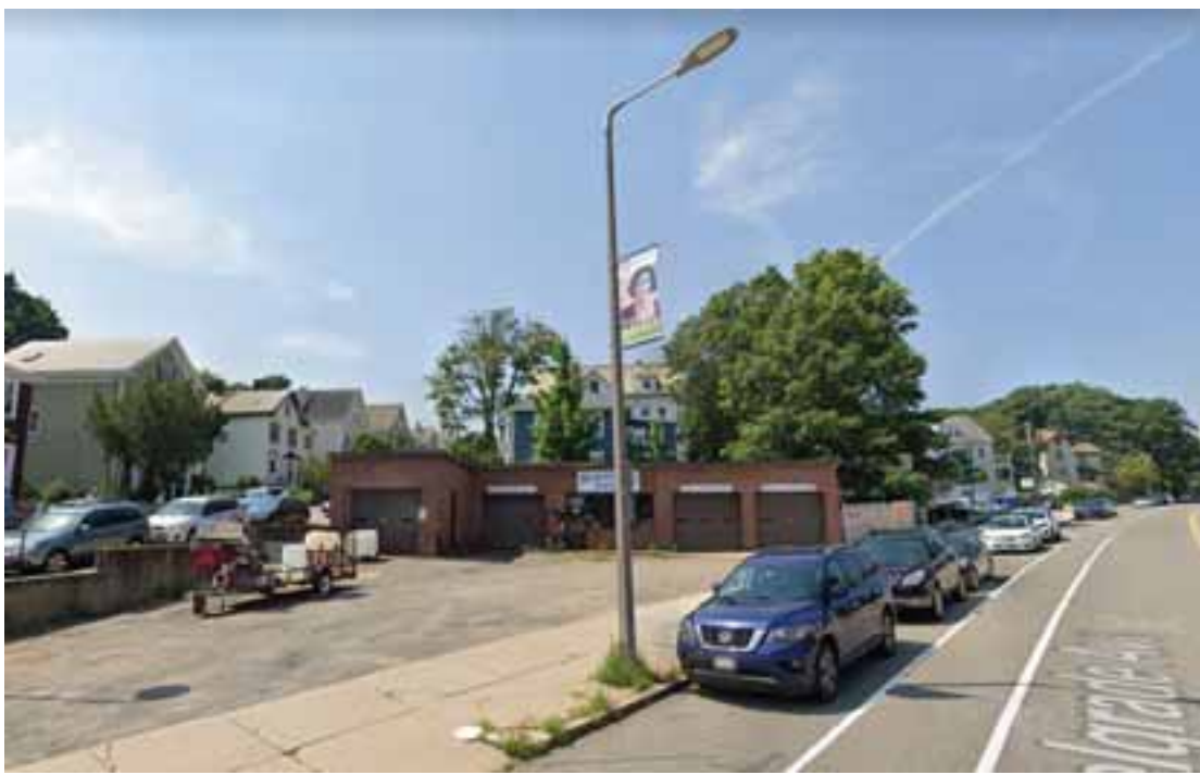
This former snow plow storage space will become home to eight condos near Roslindale Square.
