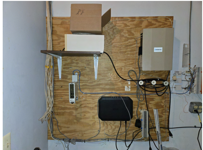
Existing network area before the new structured-cabling installation.
