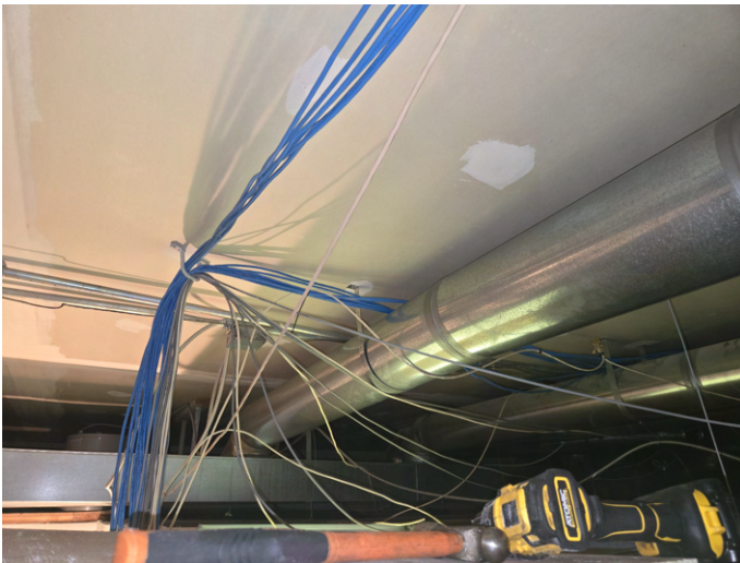
Left: CAT6 runs being routed through the office ceiling space. Right: rack, patch panels and switch installed while cable runs were being brought into the network area for termination.
