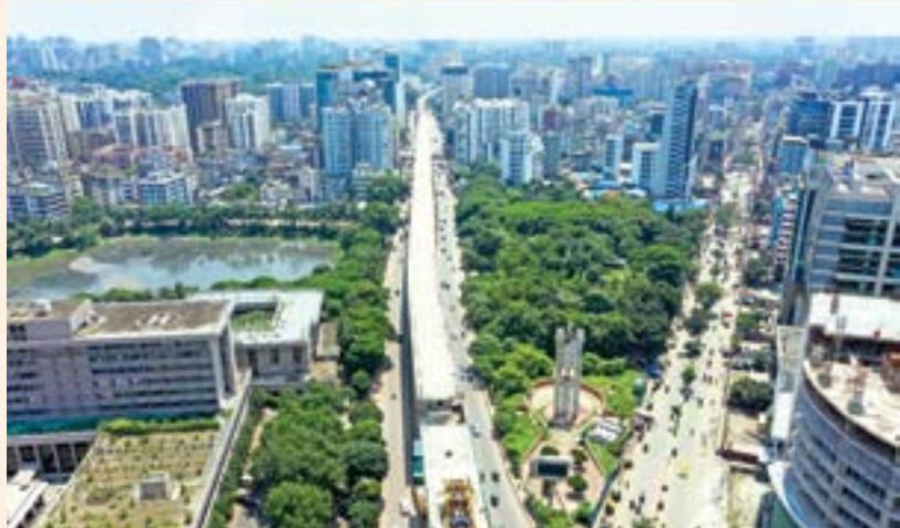
Tk 4,200 crore has been allocated in this fiscal year for MRT-6 line of the metro rail
