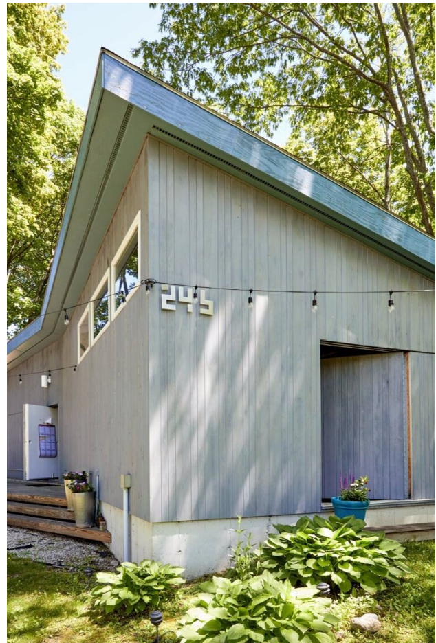
Erin and Matt built the studio in the backyard shortly after they began home renovations so that they could make use of the woodshop. The building's graceful lines were designed by Project Open. Door walls pivot outward, opening up the workshop to let the outdoors in. The exterior is composed of wood panels of varying widths that represent a bar code.
