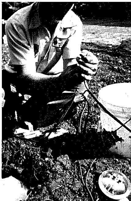
A major problem in automatic sprinkler systems is corrosion at wire connection points. To prevent this, waterproof connections should be used.
