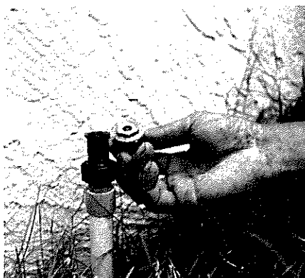
This sprinkler was causing water damage to the building because it had a full-circle head. It was replaced with a half-circle head.
