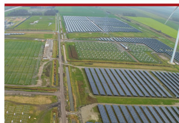
FIELD DAY: Eekerpolder solar farm under construction Photo: Novar
