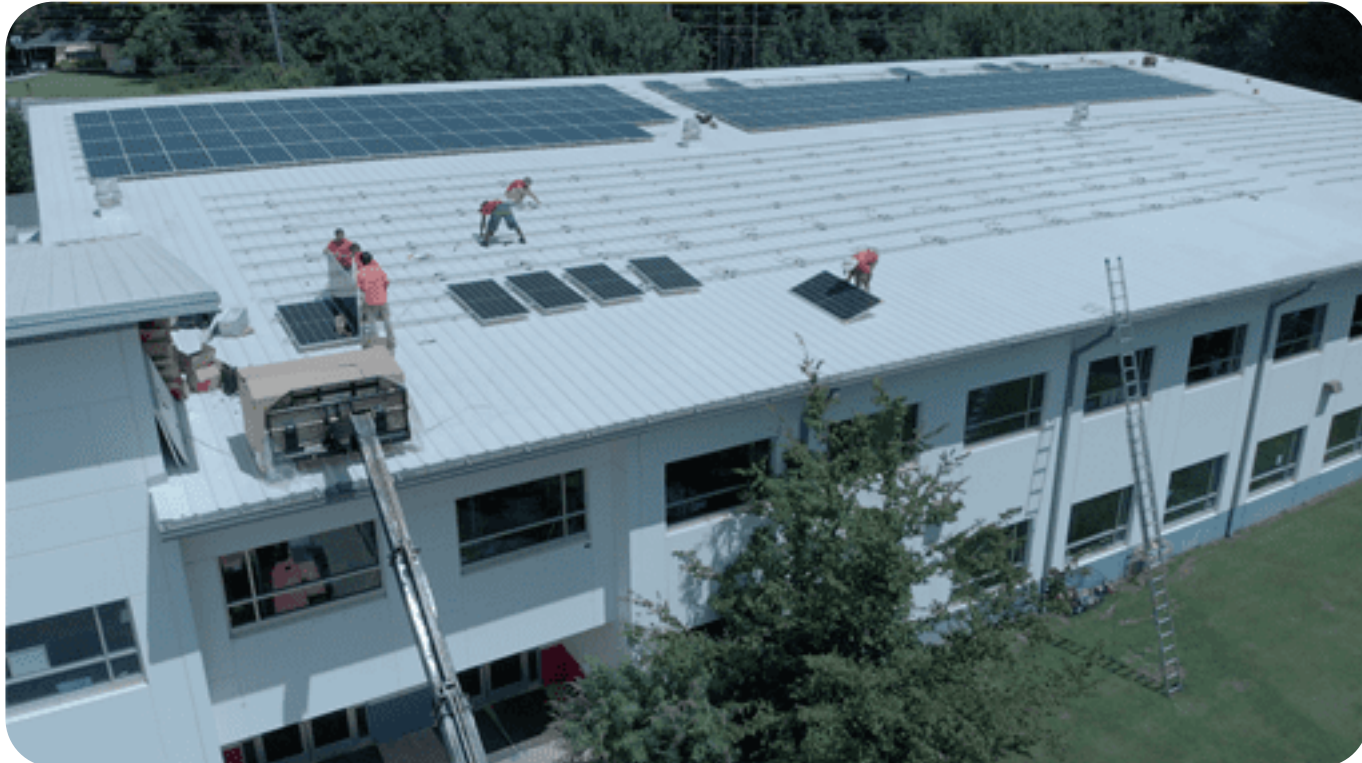
Installation of The SAE School's solar array in August. Photo by Sarah O'Connell, Creative Solar USA
