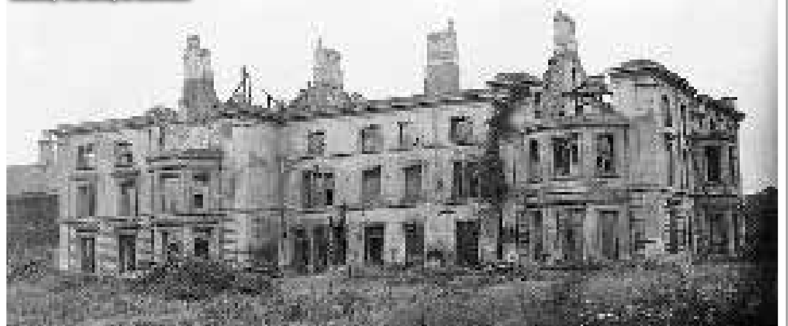
Blankney Hall during its demolition
