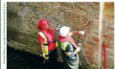
The ‘crack’ repair team
