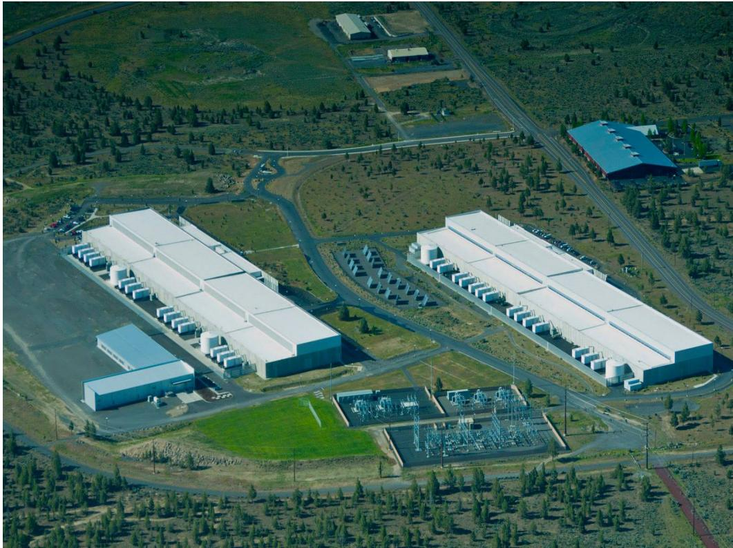
Facebook's Prineville Data Center employs an innovative evaporative cooling method that offers key advantages over the Computer Room Air Conditioning (CRAC) units in the majority of data centers. The free-air cooling system is space-saving, ultra-efficient, and quieter than other large-scale cooling solutions.
