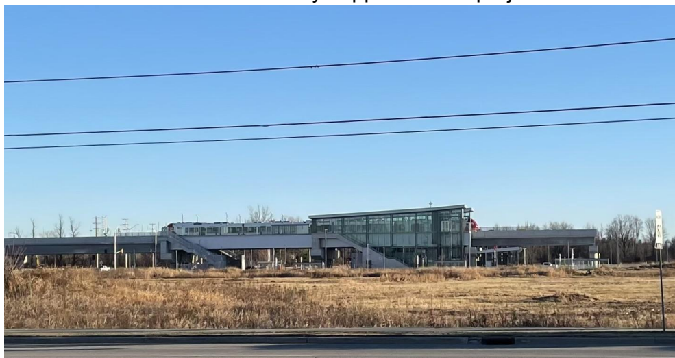
New O-Train Station on Limebank and Earl Armstrong, parallel to Armstrong Plaza
