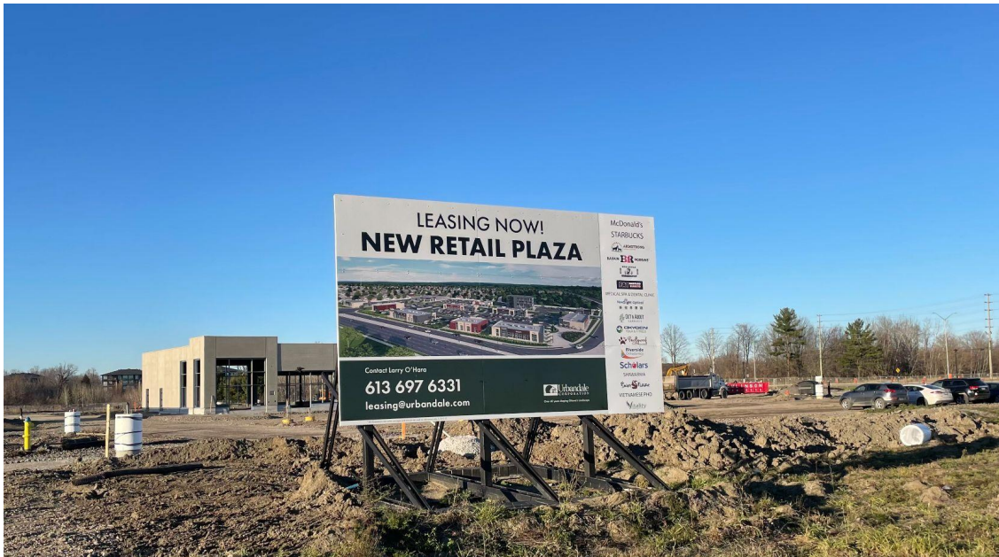
Advertisement for Armstrong Plaza with early construction surrounding
