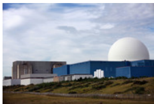
The Sizewell A, left, and B nuclear power plants operated by British Energy Group Plc., a wholly owned subsidiary of Electricite de France SA, sit on the coast in Sizewell, near Leiston, U.K. Photographer: Jason Alden/Bloomberg
