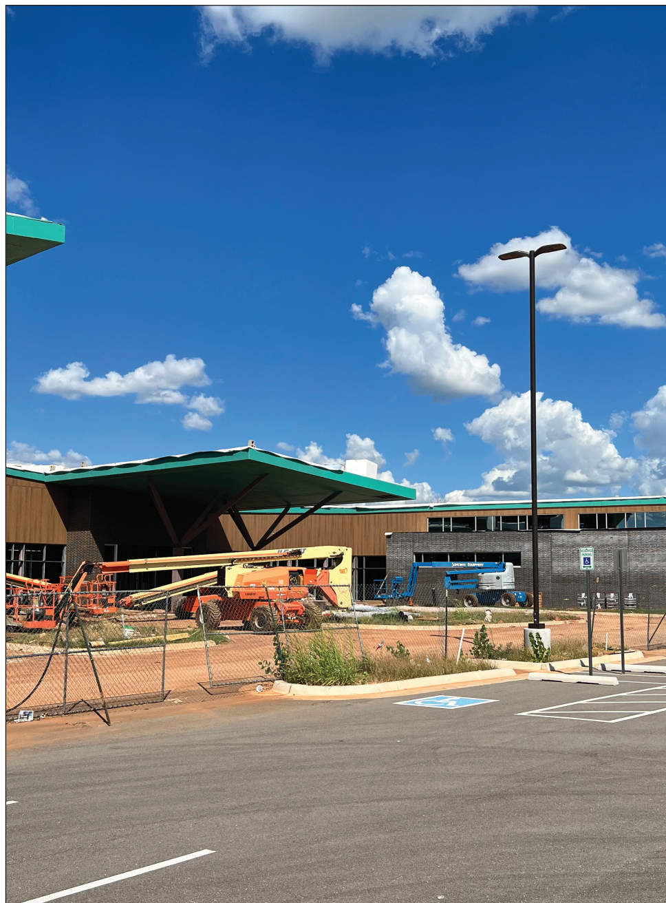
Construction of the MAPS project continues with two new senior wellness centers. (Photo by: Michael Palacios)
