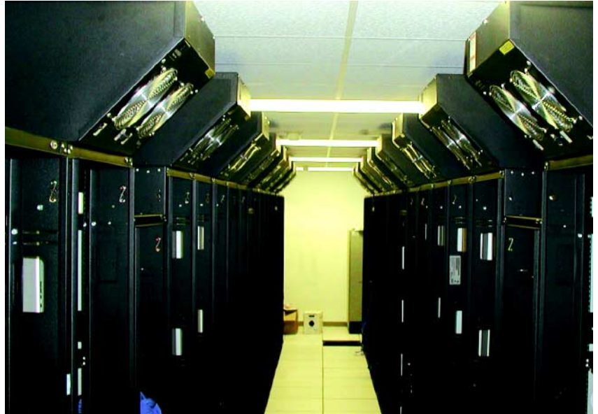
Figure 8: Supplemental cooling solutions at Virginia Tech's data center
