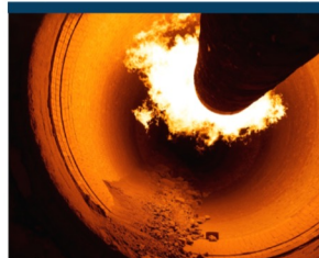
Cement and Rotary Kilns
