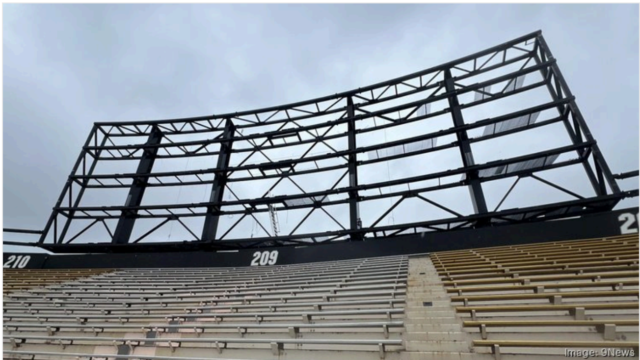
Folsom Field videoboard is under construction in April 2024.
