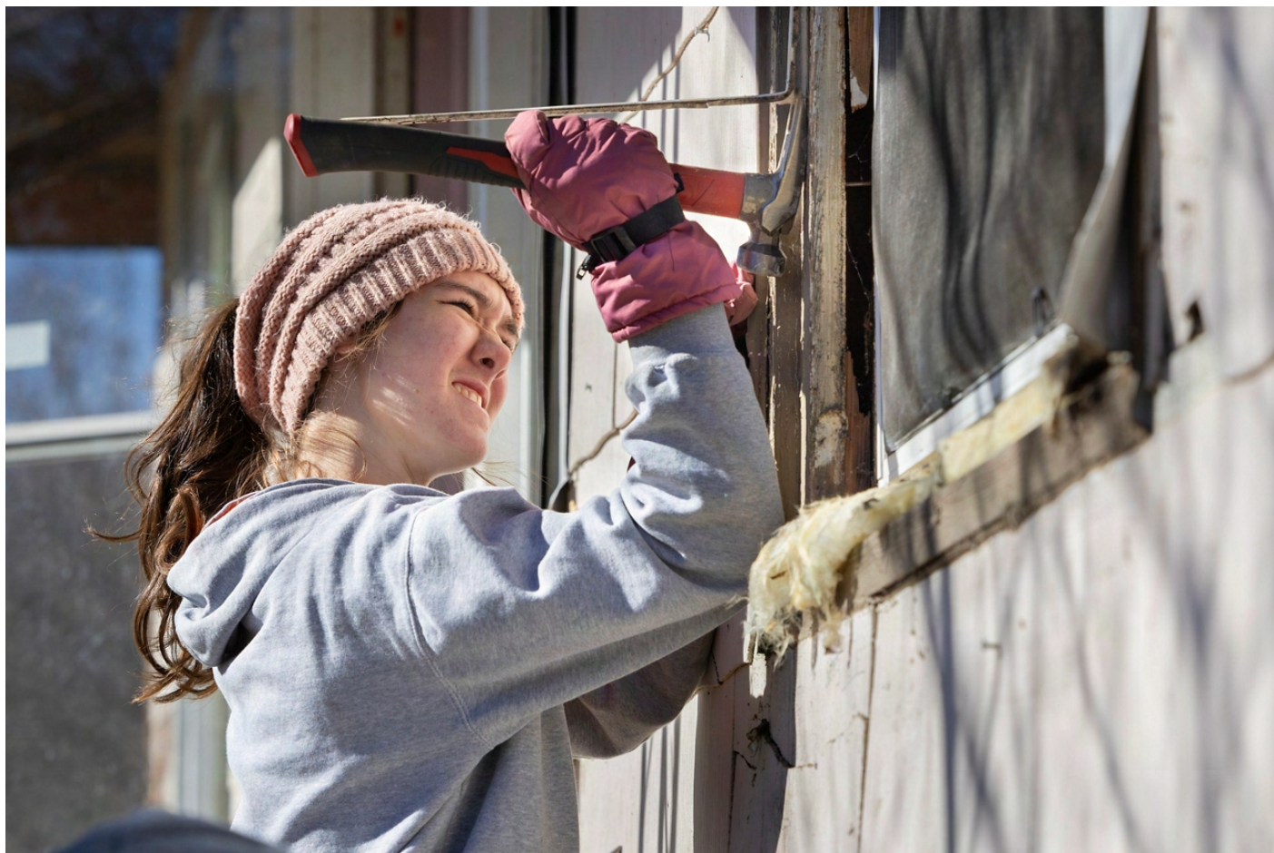
A student removes the outer layer of siding on the Hollifields' house to let moisture dry.
