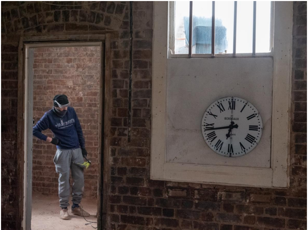
Brown's cousin Amjad Latif is cleaning the brickwork with a drill brush and sweet soap.
