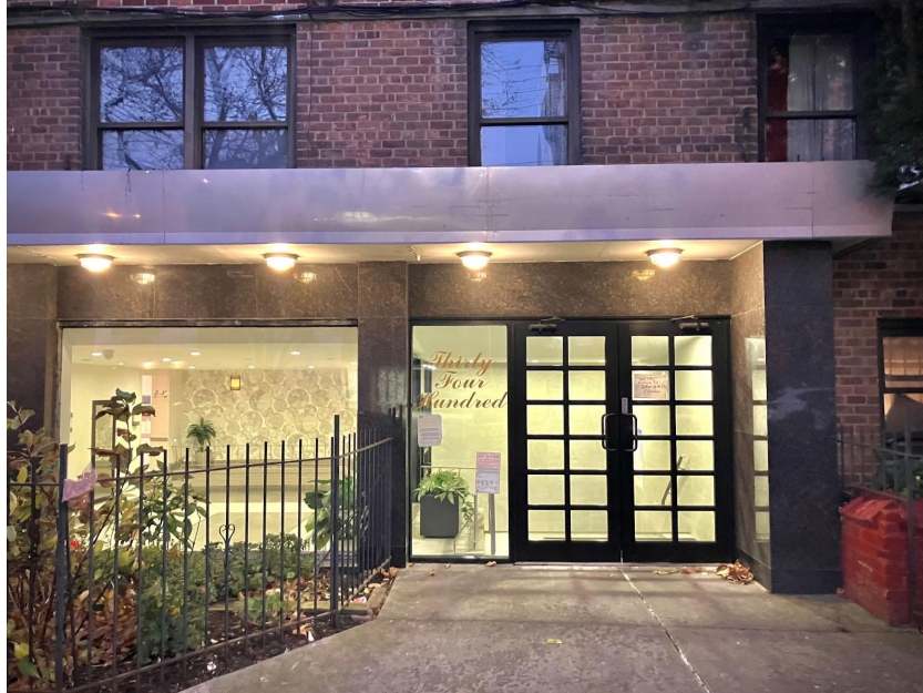
The exterior of 3400 Snyder Ave.
