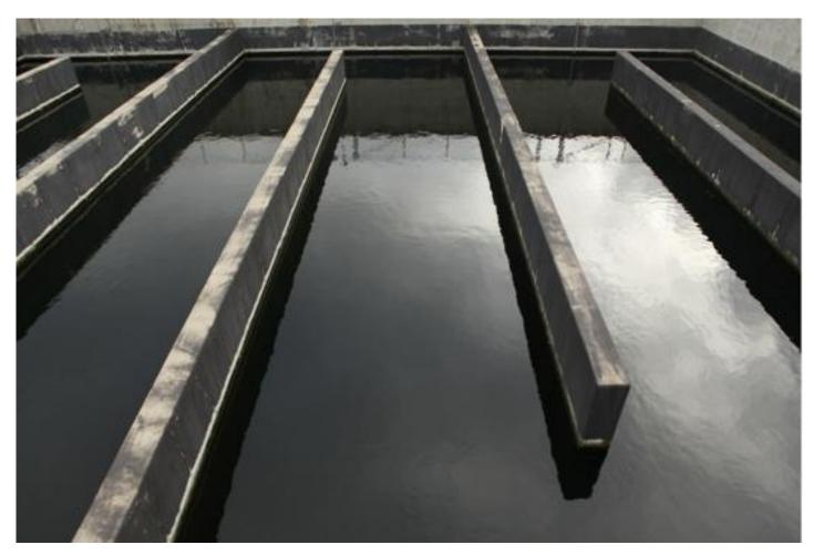
Wastewater from the southwest suburbs goes through the disinfecting tank, one of the last treatment stages before it's released into the Minnesota River, at Blue Lake Wastewater Treatment Plant in Shakopee in October 2019. The water's clean enough to swim in and even gets an added boost of oxygen for aquatic life, plant Manager Dave Simons said.
