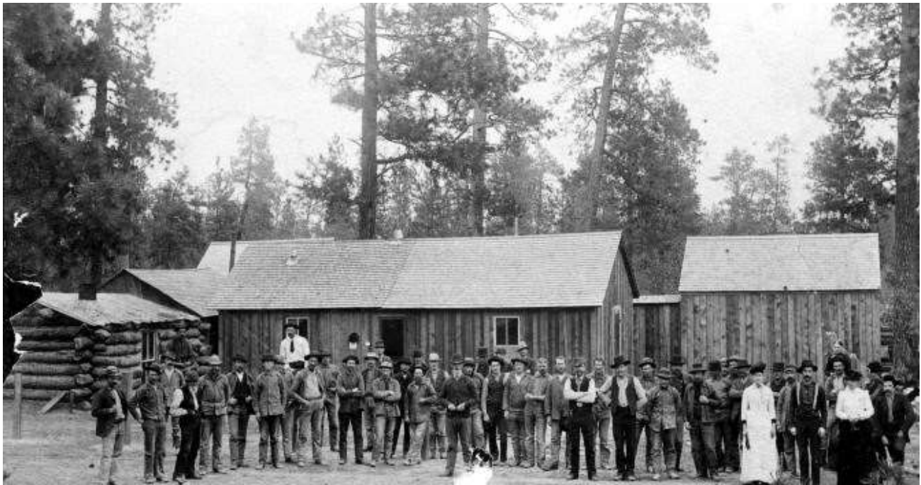
“Curlew” mine buildings (above)
