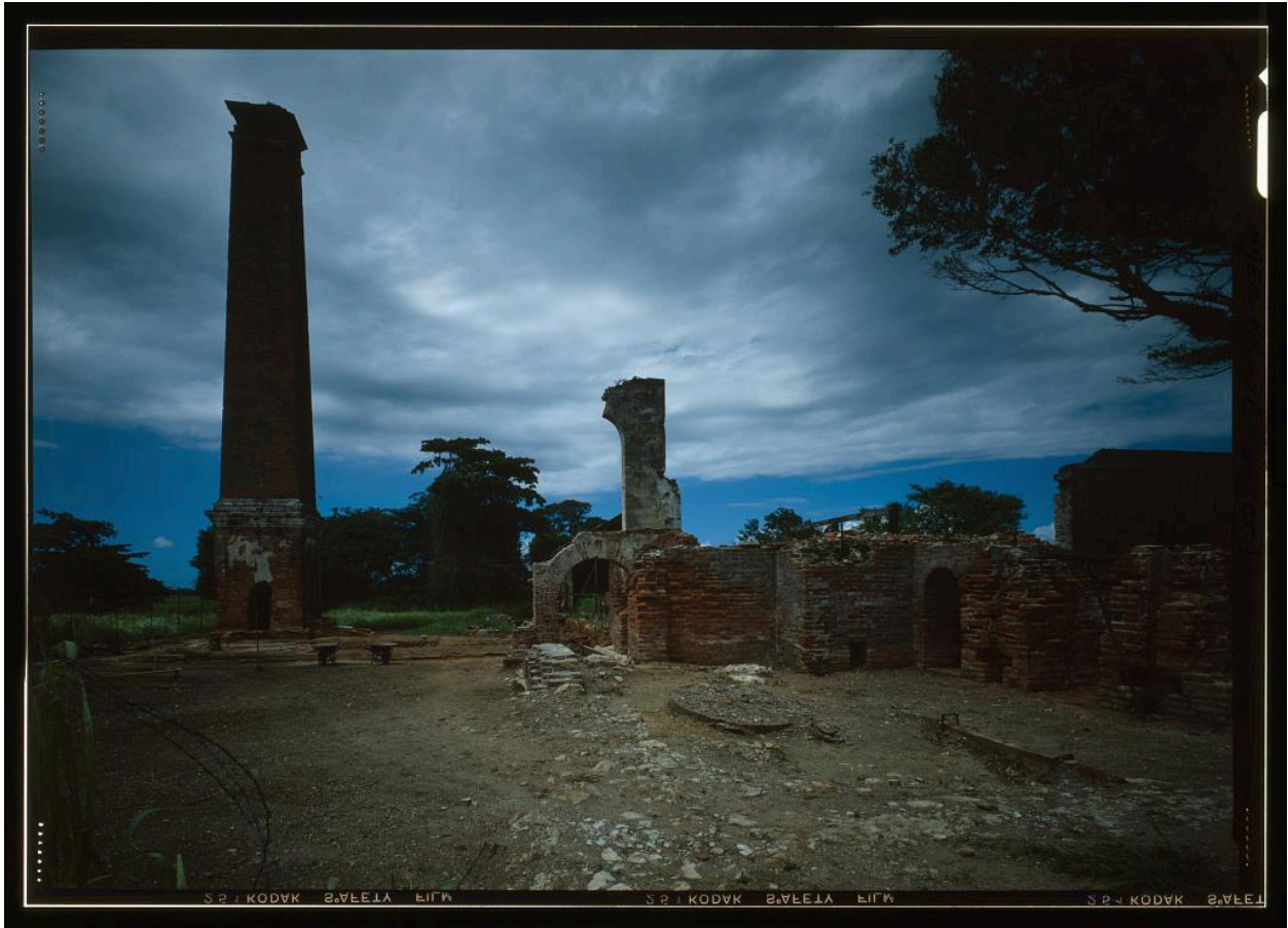
Sugar mill ruins showing chimney and masonry base of steam engine and cane mill, ca. 1968 Credit: Commons Wikipedia/ Survey HAER PR-1-B Historic American Engineering Record
