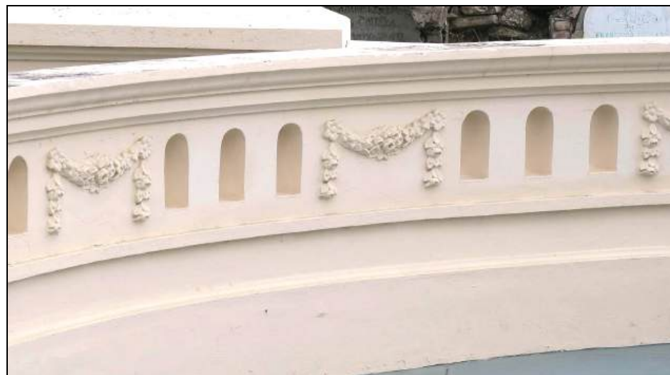
Wall detail, left side of Mausoleum, 2024
